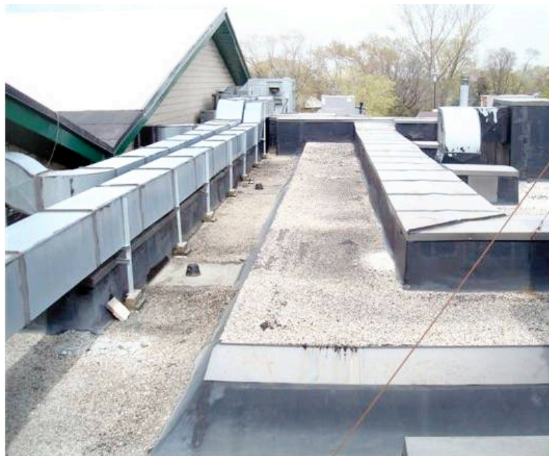
Before Eco-Roof installation
